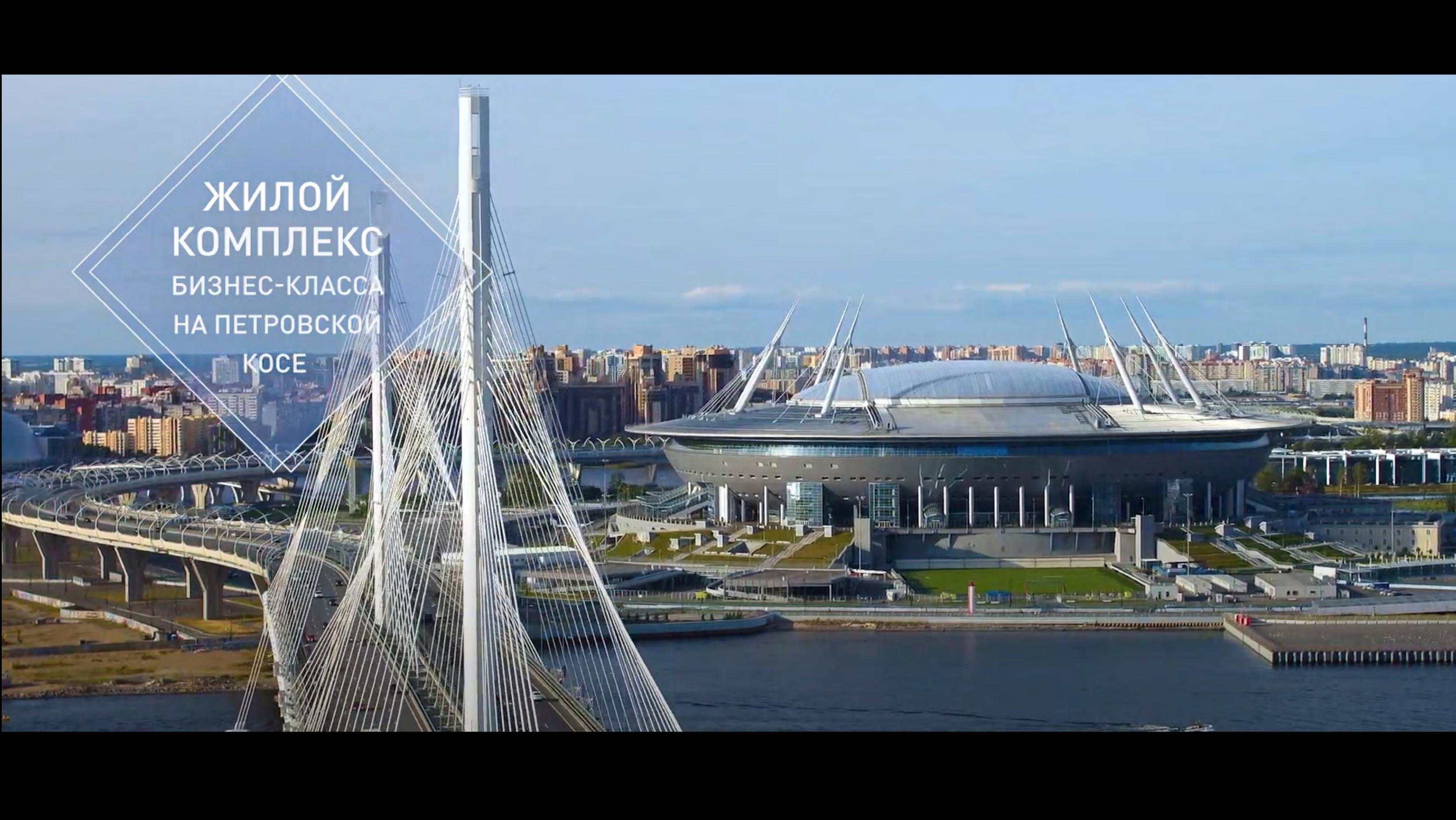
An aerial photograph showing a modern cable-stayed bridge in the foreground, with a large, futuristic stadium in the middle ground. The stadium has a distinctive white, ribbed roof and is surrounded by a cityscape. The bridge's white cables fan out from a central pylon. The stadium's roof is supported by several tall, white, angled masts. The city in the background consists of numerous multi-story residential buildings. The sky is a clear, pale blue.
